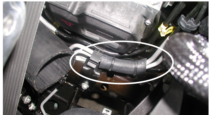
Insulation Onto Brakeline Installed
